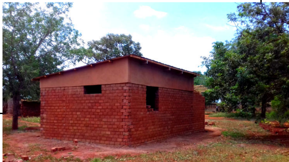
Construction at different phases.
