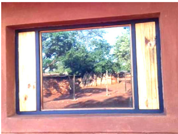
Views of windows with shutters (made with reclaimed wooden pallets and grass roll-up blinds).
