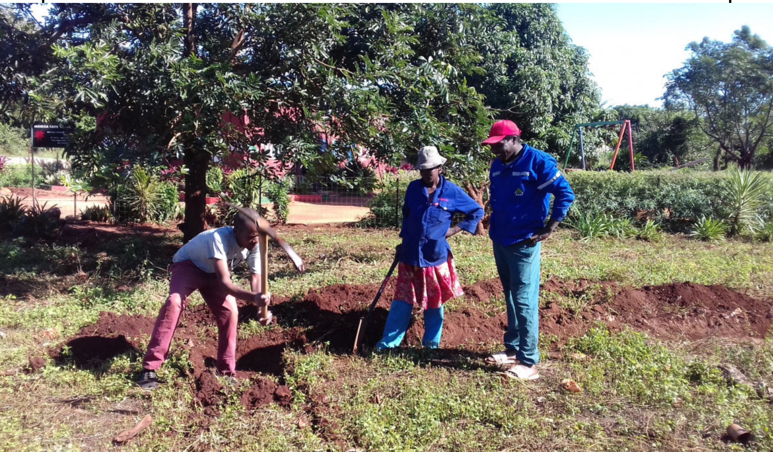
Digging of the house's foundation trench.
