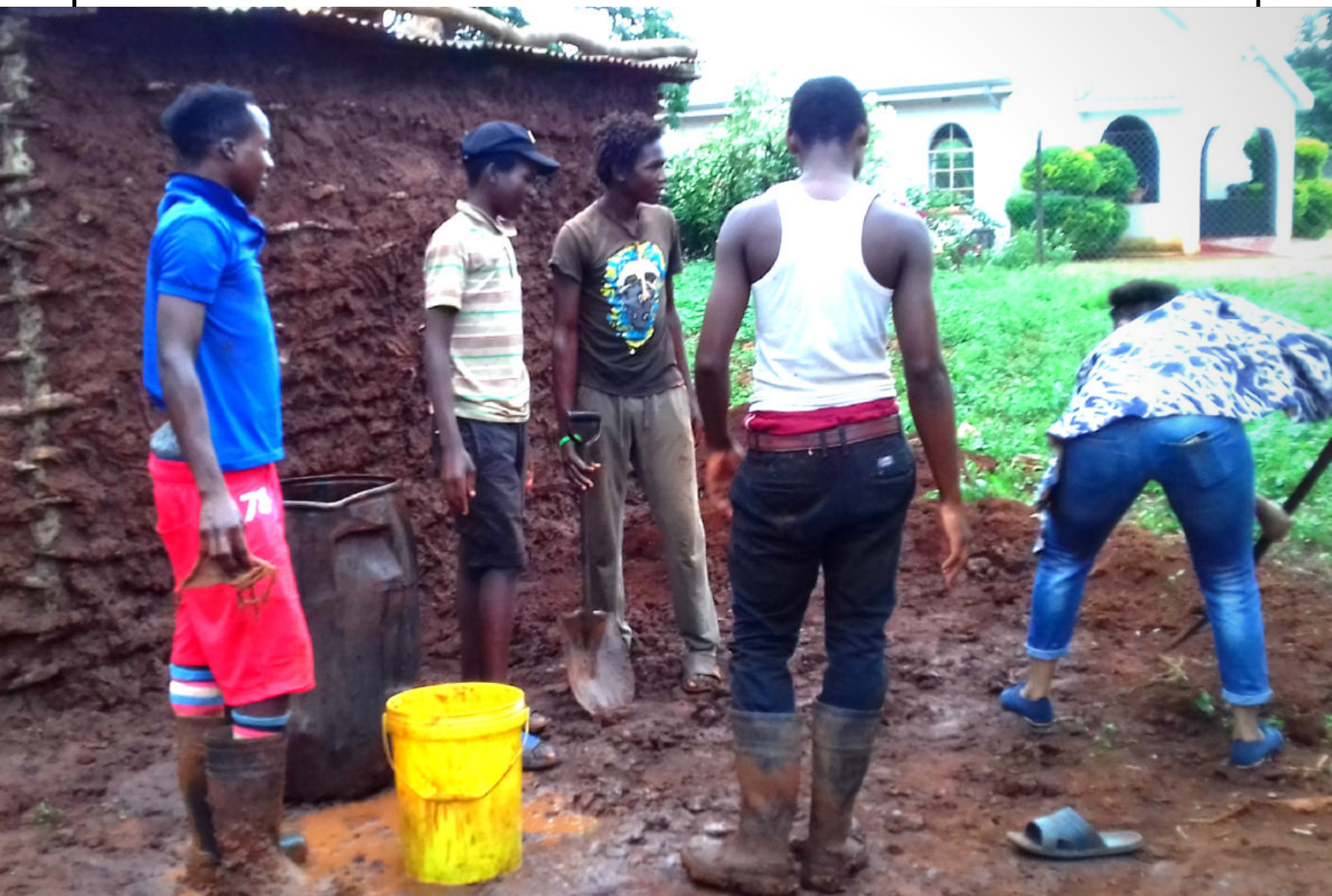
Mgidza residents creating mud to plaster the current housing's sticks and stones.
